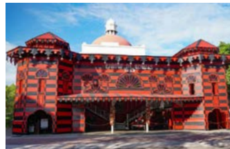
Parque de Bombas in Ponce.
